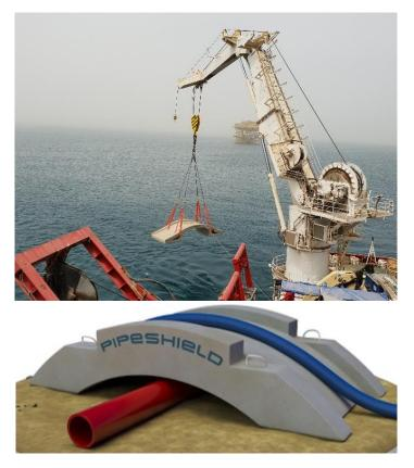
*Figure 3.19. Method for constructing and laying concrete structures on a cable line (source: www.pipeshield.com/products/concrete-structures)*
