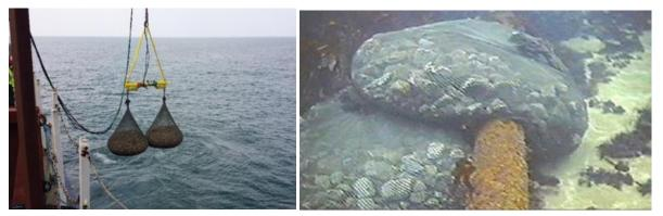
Figure 3.18. Method for constructing and laying rock bags on a cable line (source: www.bluemont.com.au/erosion/kyowa-rock-filter-bags/offshore-subsea)
