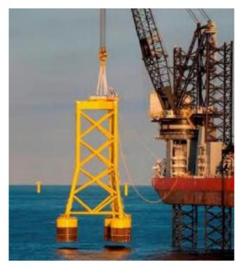
Figure 3.7. Example of a Suction Bucket (Caisson) Jacket Foundation [source: DNV report "Assessment of Offshore Wind Farm Decommissioning Requirements"]
